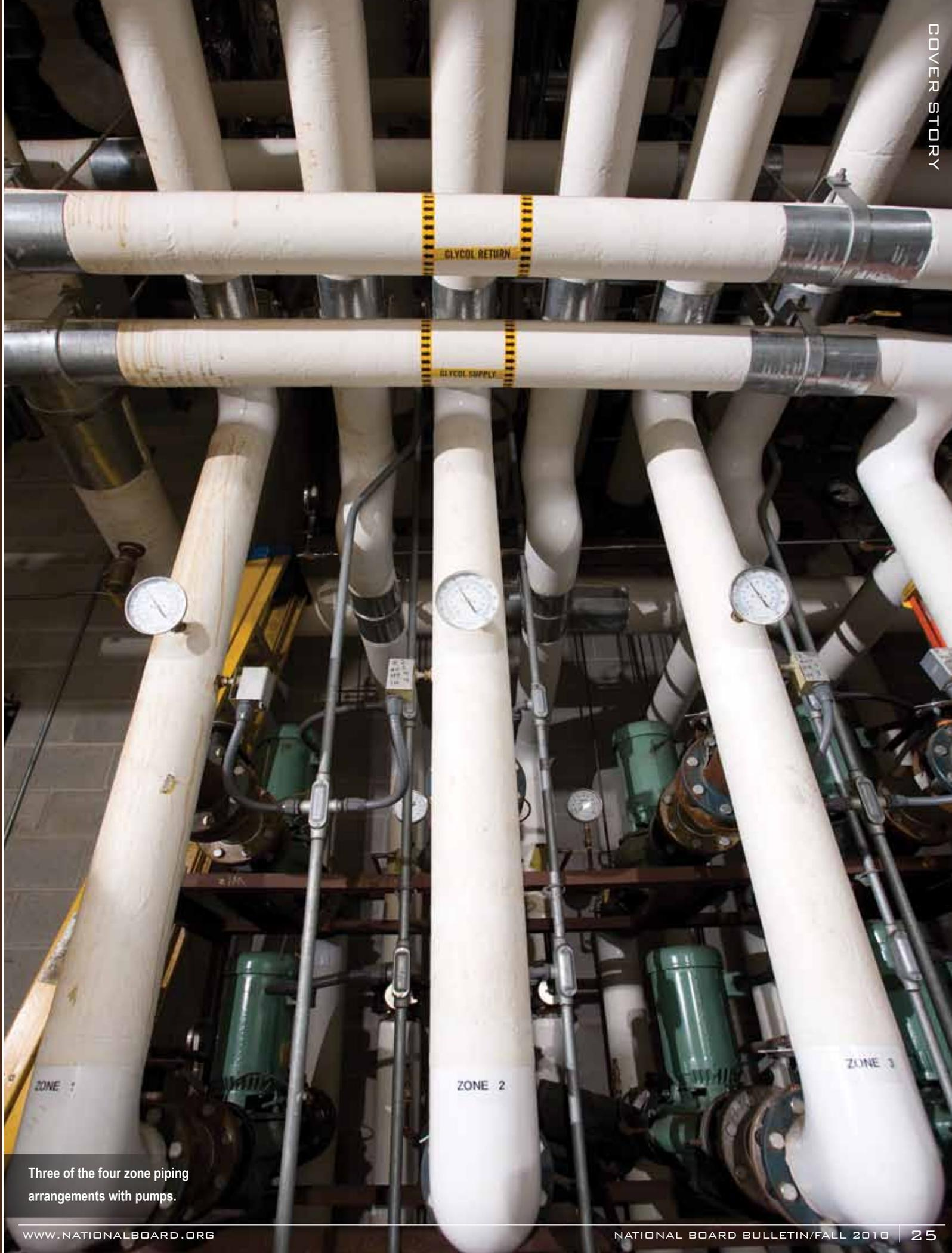
Three of the four zone piping arrangements with pumps.
